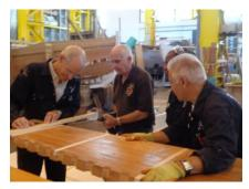
Finally having completed the holes it was time to glue up both sets of engine bearer. Middle photo below Steve B is putting the glue onto all of the surfaces and below right he and John S are clamping up the joints having first aligned the critical water line to make sure that we didn't have any unplanned bendy bits in the hull
