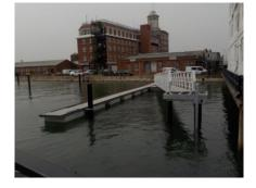
month, below left some of the pontoons are being prepared ashore on the sliway before floating them round the the dolphins. Just to the left the dolphins are in place and the first sets of pontoons are connected up along with an access gangway. This new arrangement will allow for
