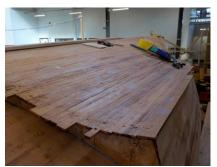
the trailing edge of the step and over left shows the port side as the planking is progressed by the other teams . At this stage the planks have not been faired down but the trailing edge has been screwed to the former, the twin rows of screws can just be seen.
